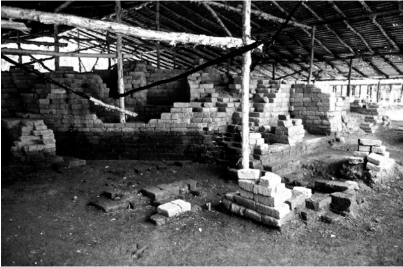
Fig. 19-12: Candi 3 under restoration at Bumiayu (Photo: EFEO)
